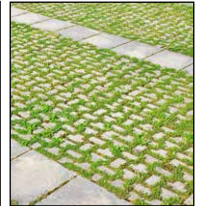
Figure 89: Permeable paving. (Photo © Adobe Stock 2022)
