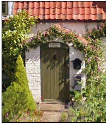
F.40: Brick built porch with pantiled roof. (Photo © Google Earth 2022)
