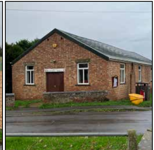
F.64: Parish hall. (Photo © AECOM 2022).
