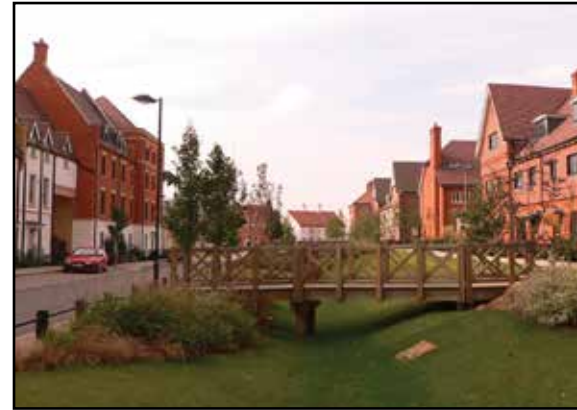
Figure 88: Example of open drainage channels. (Photo © AECOM 2022)
