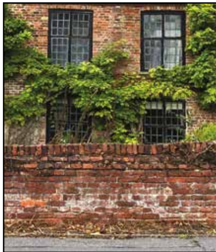
F.43: Traditional leaded windows. (Photo © AECOM 2022)
