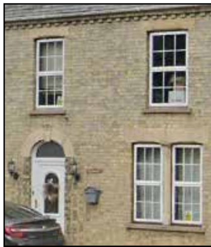
F.45: Georgian house with sash windows. (Photo © Google Earth 2022)
